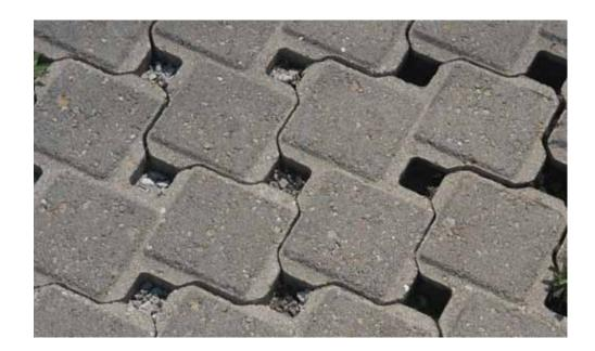
Porous surfaces can be thought of as a rigid, load bearing area with an internal structure not unlike open cell foam. When water comes in contact with the upper surface, it flows immediately through the surface to the engineered volume under it.
